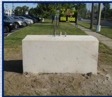
Concrete & Civil Work
