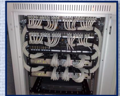
Data Cabling & Works
