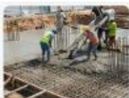
Concrete & Civil Work
