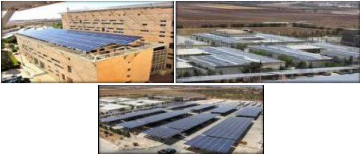
2.11 MW PV PLANT – GERMAN JORDANIAN UNIVERSITY
