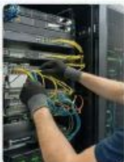
Data Cabling & Data Works
