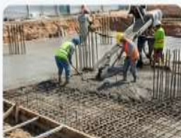
Concrete & Civil Work
