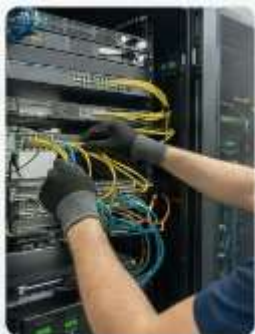
Data Cabling & Data Works
