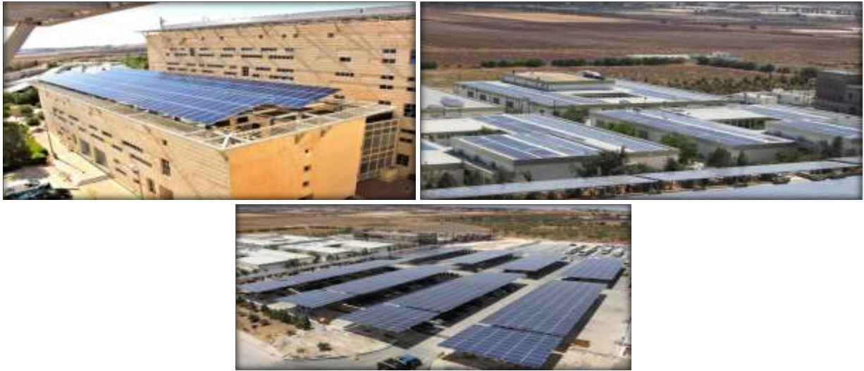
2.11 MW PV PLANT – GERMAN JORDANIAN UNIVERSITY
