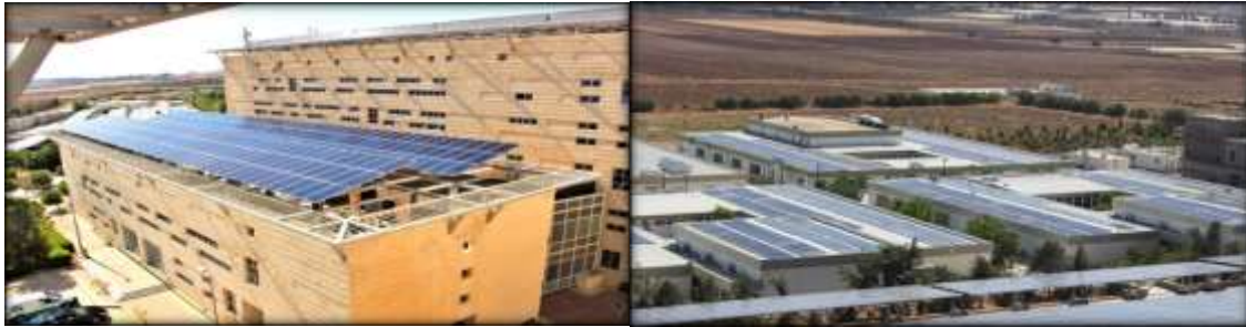
Rooftop Solar Systems
