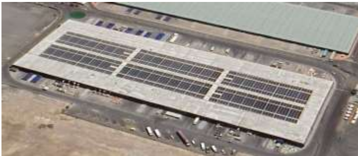
1.75 MW PV PLANT – AMAZON WAREHOUSE, JEDDAH – KSA
