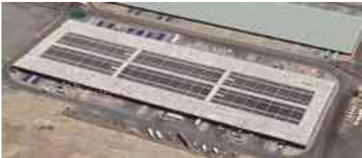
1.75 MW PV PLANT – AMAZON WAREHOUSE, JEDDAH – KSA
