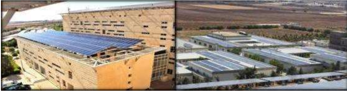
Rooftop Solar Systems
