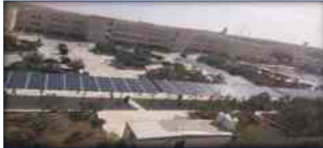
5 MW PV PLANT – HASHEMITE UNIVERSITY
