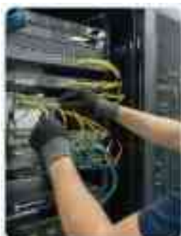
Data Cabling & Data Works
